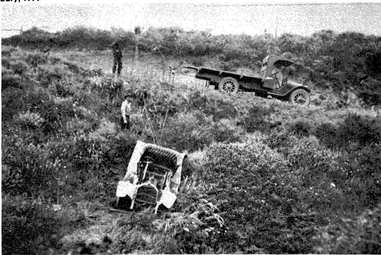
A RESCUE OF THE PAST. It is believed that one of the rescuers pictured is J.W. Post Jr., "The Ol' Master."
