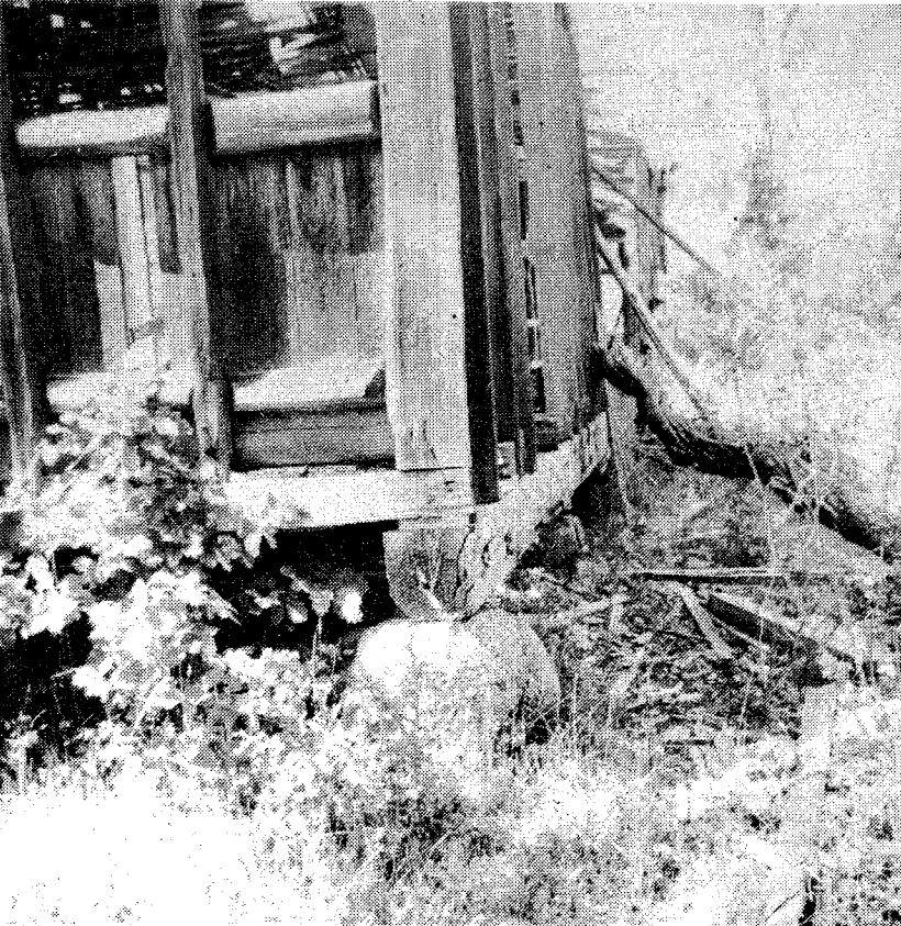
CLOSE UP of the ranch house foundation today -- held by stone for more than 100 years.
